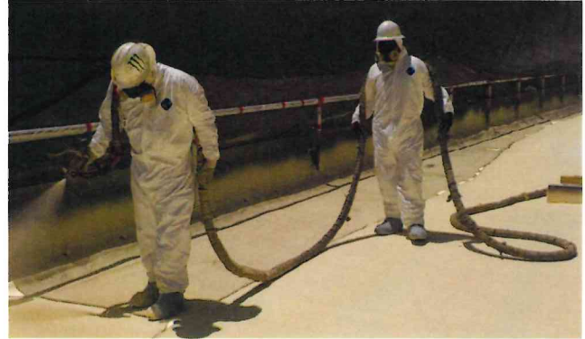
Application of SPF on a low-slope roof.
