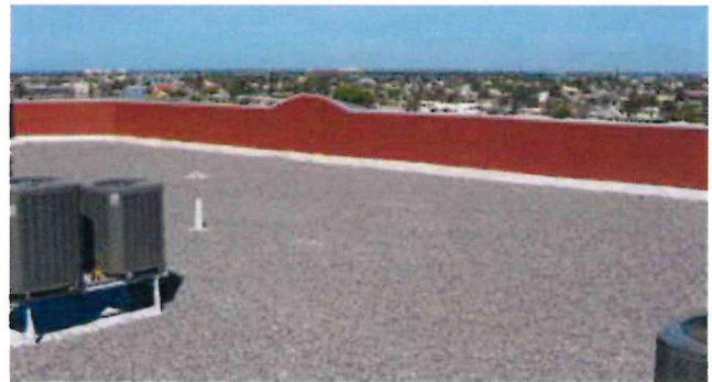
Application of SPF followed by an aggregate covering.
