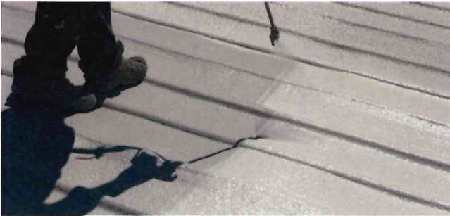
Application of SPF over a metal roof followed by an acrylic coating.
