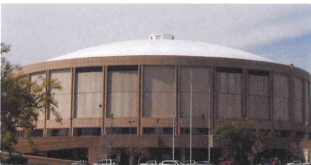
The SPF roof on the Biloxi (MS) Coliseum survived 12 hurricanes since 1979.
